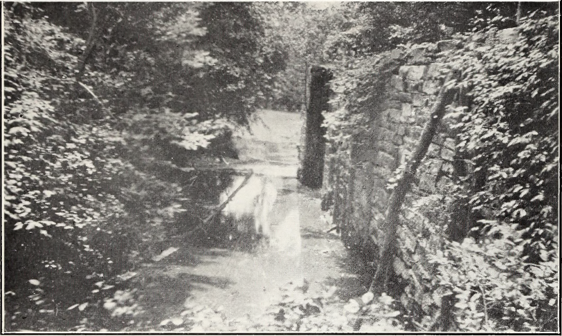
Old Lock, now foundation of power house, Moncure
